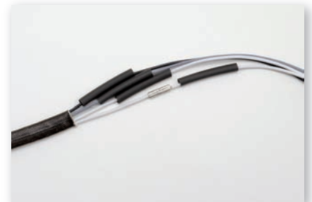
Slide the heat shrink tubes until is over the butt-type connector
